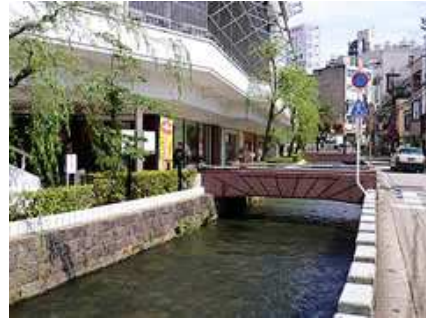
The uncovered channel of the Kuratsuki Canal
