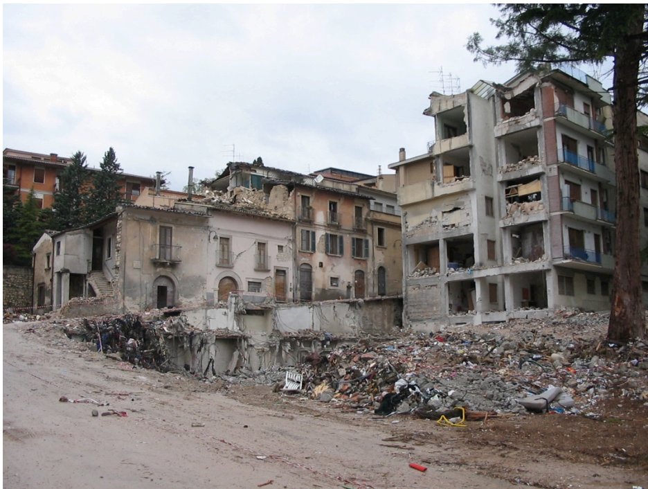
Figure 12 Residential neighborhood, downtown L'Aquila, 2009
