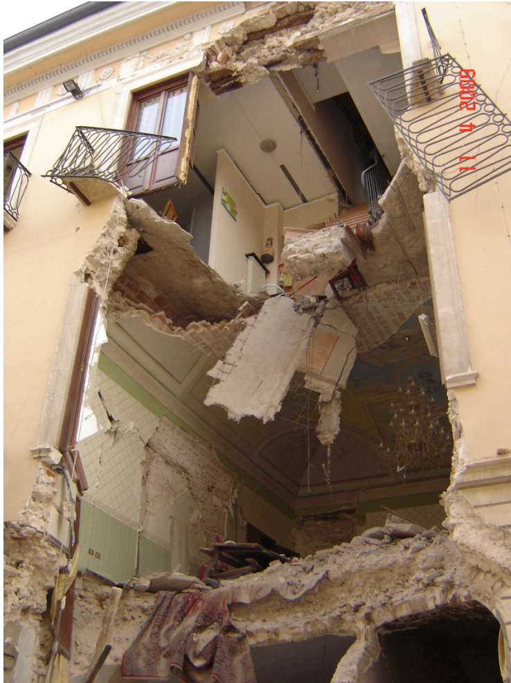
Figure 15 Collapsed apartments in the UnivAQ neighborhood, 2009.
