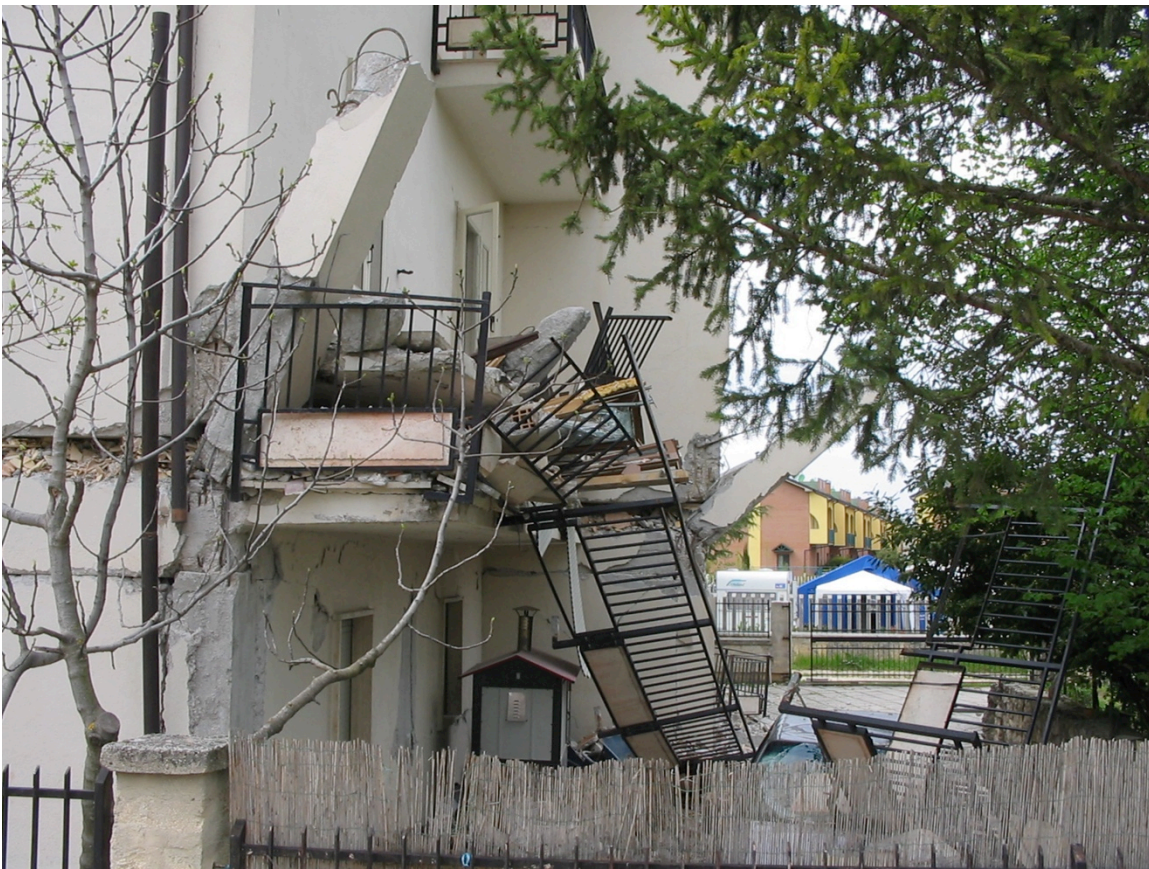
Figure 17 My neighbor's house, middle story collapsed, L'Aquila, 2009.
