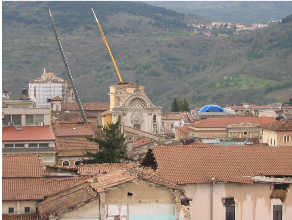
Figure 5 View of the roofs of downtown L'Aquila, 2009.
