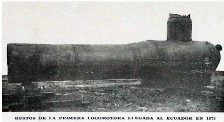
The surviving boiler of no. 1 , as photographed in 1933. Note the very shallow firebox.
