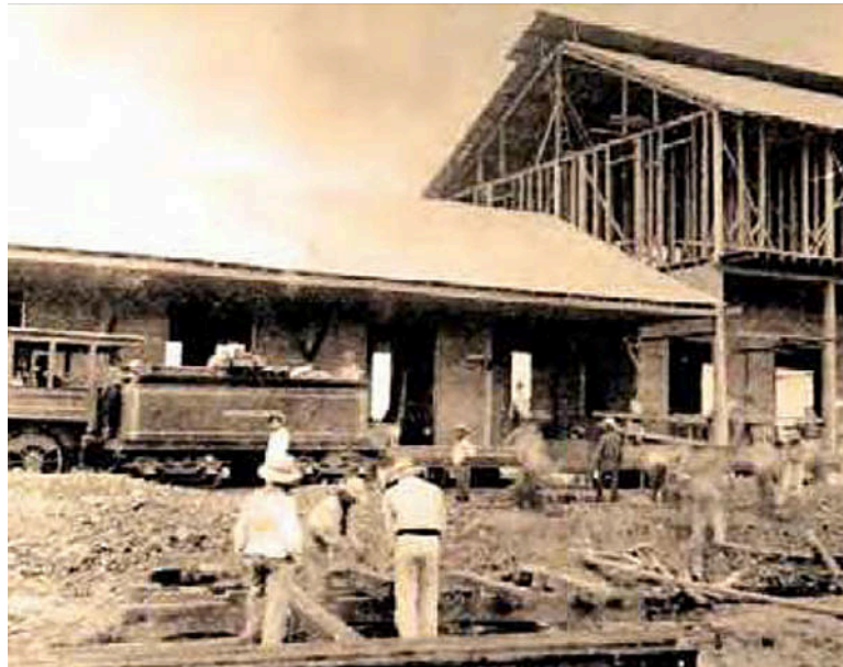
This photo shows the big station building at Durán under construction. The loco partially visible on the left would seem to be the Grant 4-4-0 illustrated above.
