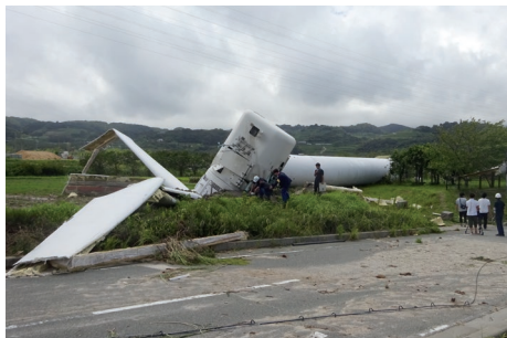
Collapsed wind turbine in Awaji City, Hyogo Prefecture (Due to a typhoon in August 2018)
