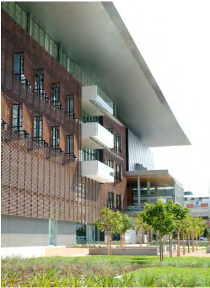
Fig. 3 Gallery of Modern Art, Brisbane. The Western façade, showing timber screening. Architectus and Davenport Campbell in association. Completed 2005. Photograph by John Macarthur, 2013, used with thanks.
