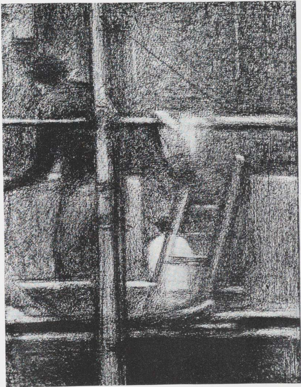
125 Scaffolding. Anonymous loan
