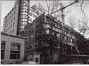
Ducat 2 office building, Moscow, under construction, Liebman Melting Partnership
