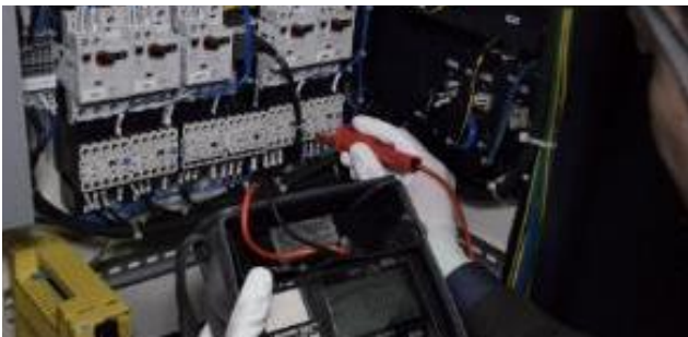
Measurement using megohmmeters (once/year)
