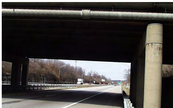
Figure 7 Existing 12" Water Main over I-264
