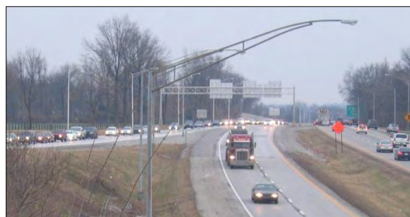
Figure 2 Exit ramp queues back up onto I-264.
