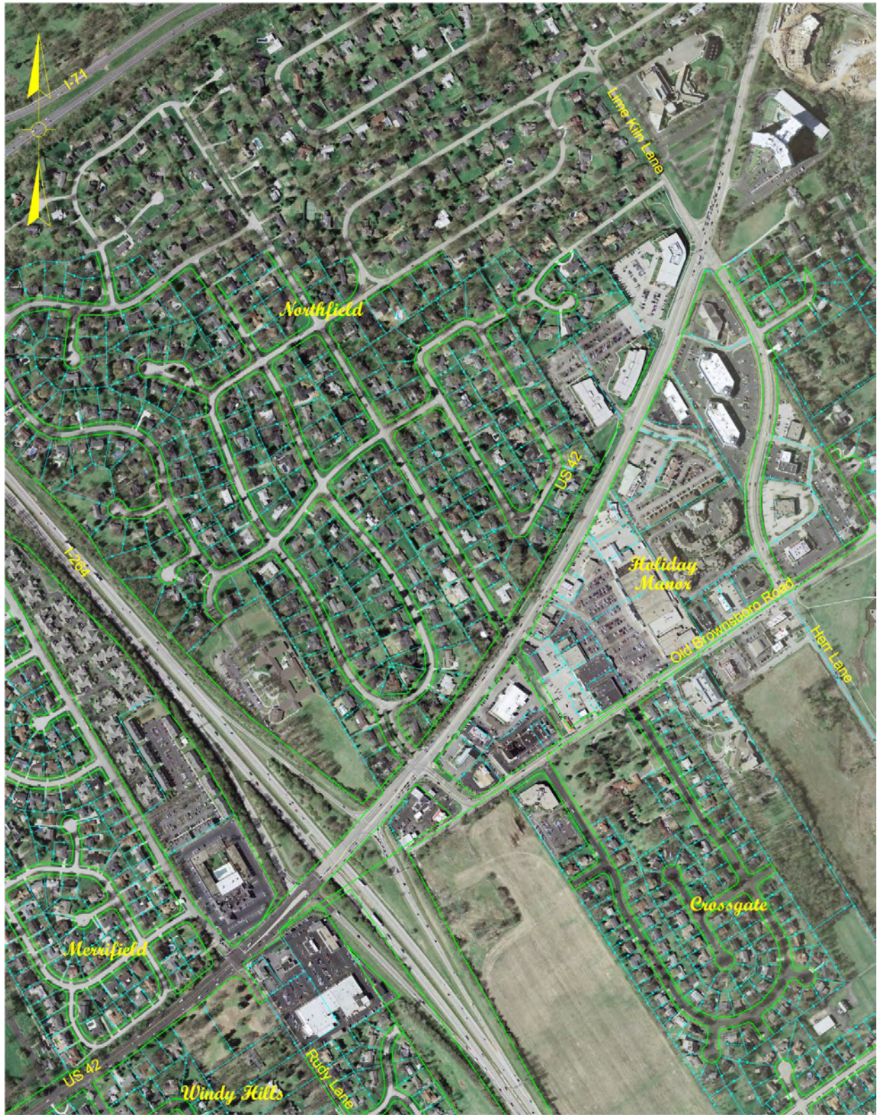
Figure 8--Existing Right of Way
