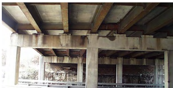
Figure 6 Existing Structure over I-264
