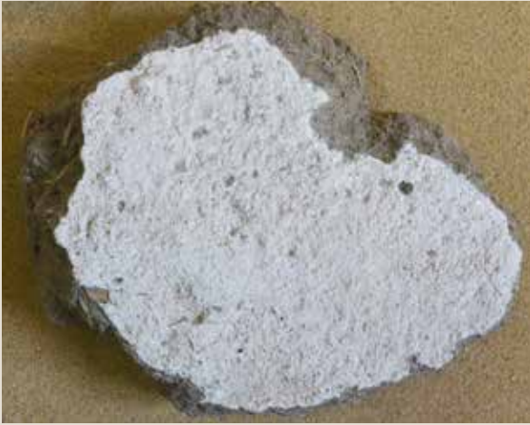
PL153. From KRO, thick pure white paint applied over grayish-brown plaster with cut straw and pebbles. The surface is rough flat alluvial mud, with tiny cavities in it. In contrast to other white paint used at Giza, this one is especially white, probably because it contains a high percentage of gypsum.
