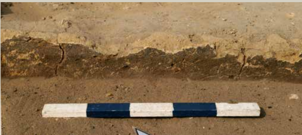
Dado. Traces of a dado on the wall in situ in House Unit 1 at HeG. The grayish-black layer (3 millimeters thick) was applied over a thin layer of white painted plaster, which was applied over yellow marl clay.
