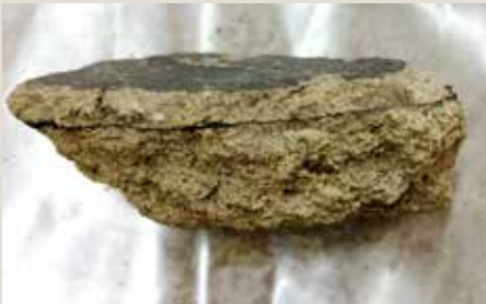
Plaster repair. This is one of only two examples of wall plaster that had been repaired. A layer of black-painted plaster was applied over an older layer of black-painted plaster. Both examples had been applied over mud plaster.
