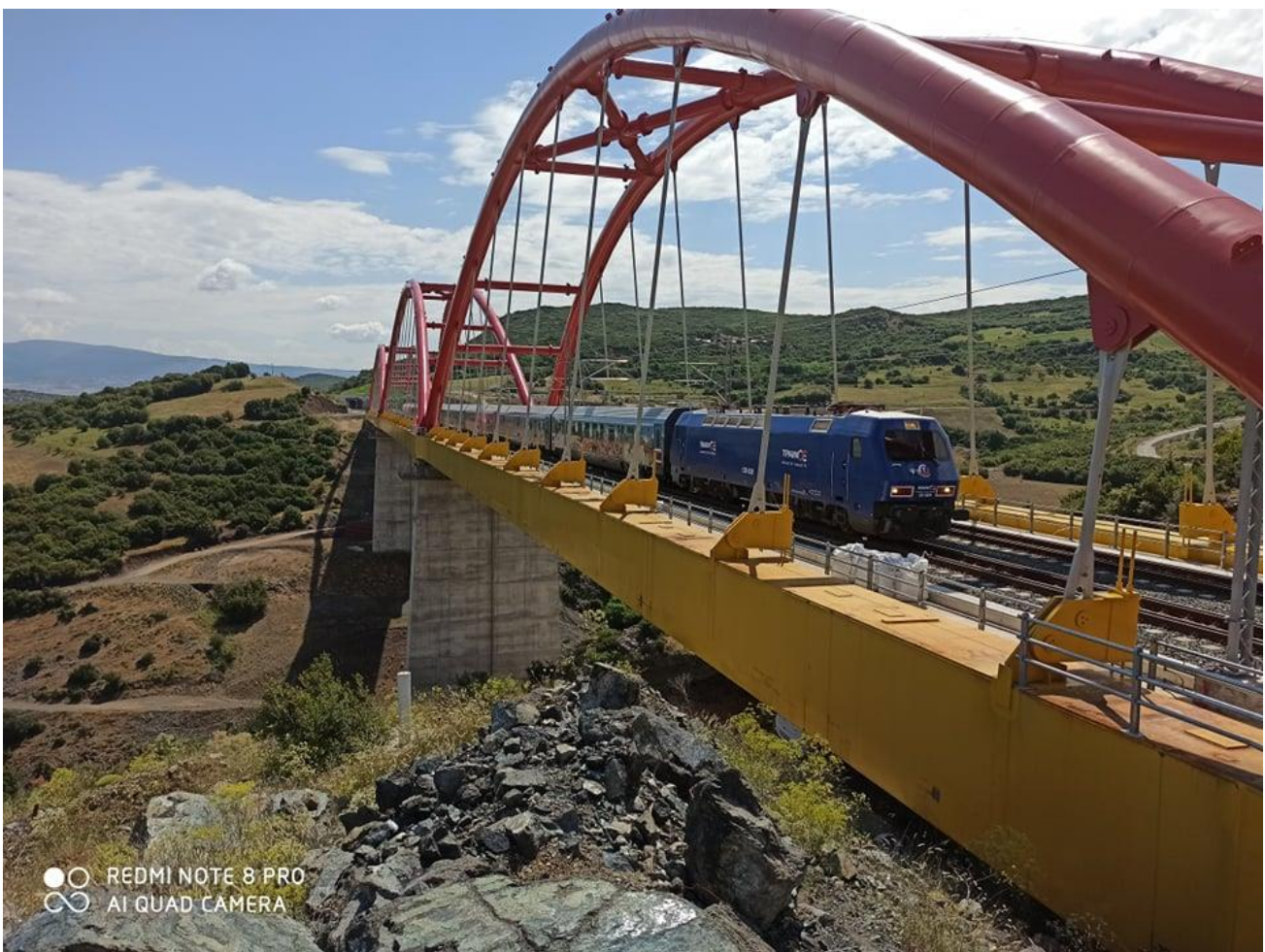
Railway Bridge RB26, in Domokos, completed in 2018 (as part of Action 2014-EL-TMC-0651-W). Source: ERGOSE S.A.
