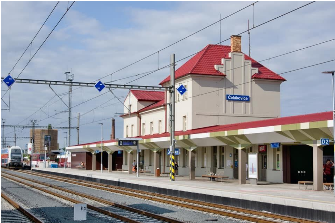
Works completed at Čelákovice railway station (2016-CZ-TMC-0014-W). Source: Správa železnic
