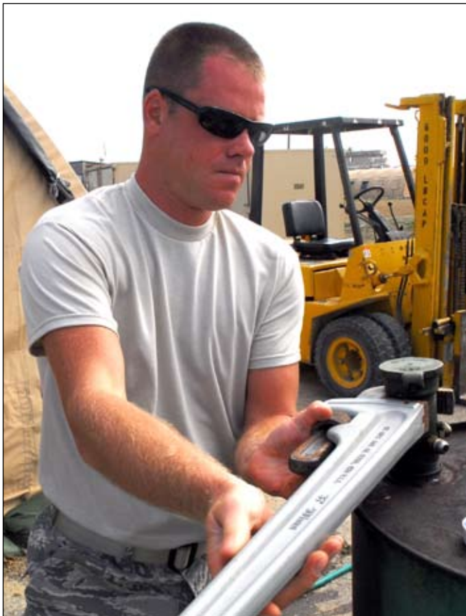
Air Force Senior Airman Ryan McClung works on a boiler. – JTF Guantanamo photo by Army Sgt. Michael Baltz
